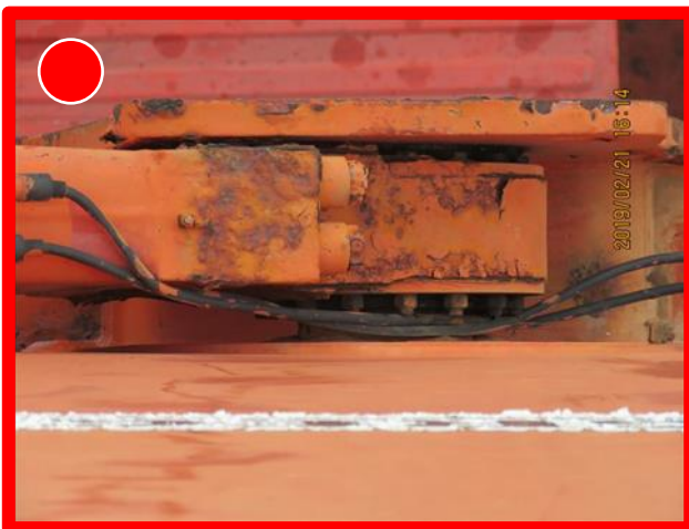
Excessive corrosion on jib mounting
