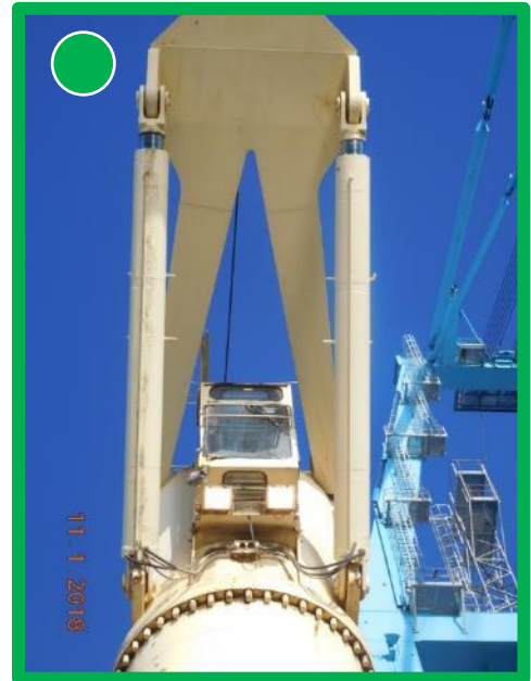
Luffing cylinders sound, no corrosion
