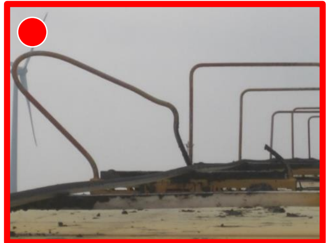
Distorted wire jumper
