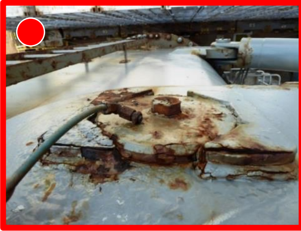
Jib pivot point / hinge pin with excessive corrosion
