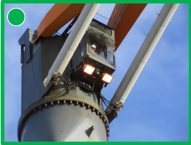
Luffing cylinders sound, no corrosion
