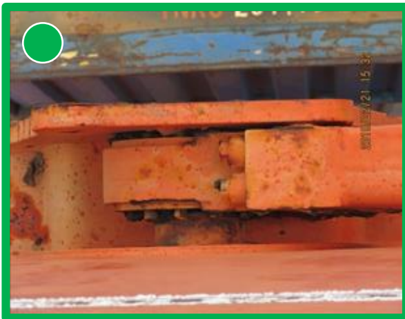
Progressive corrosion on jib mounting
