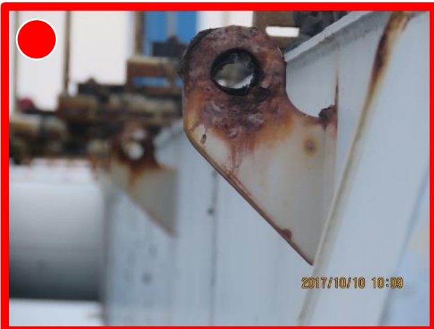
Lifting eyes on jib with excessive corrosion
