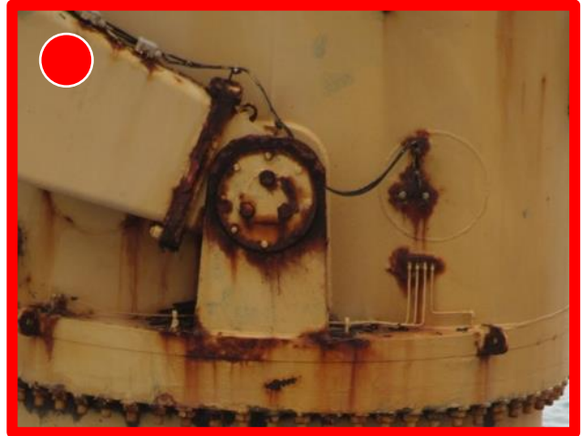
Jib hinge with excessive corrosion (also on slewing ring)
