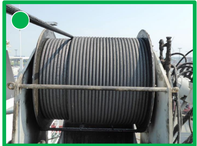
Wire drum with minor, progressing rust
