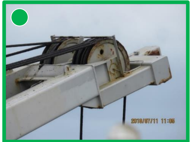
Jib end sheave with progressive corrosion
