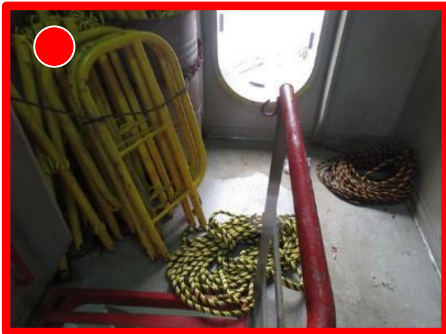
Pedestal entrance with objects obstructing passage
