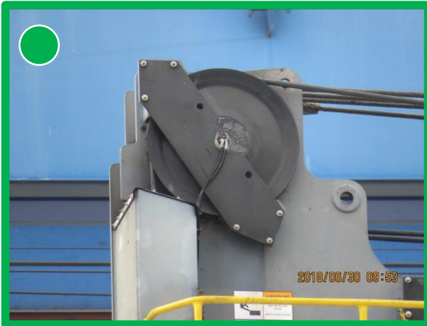
Crane top wire sheave, sound
