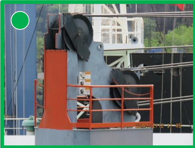
Topside handrailing sound
