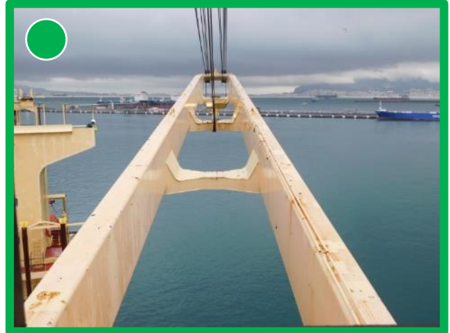
Superficial corrosion on jib
