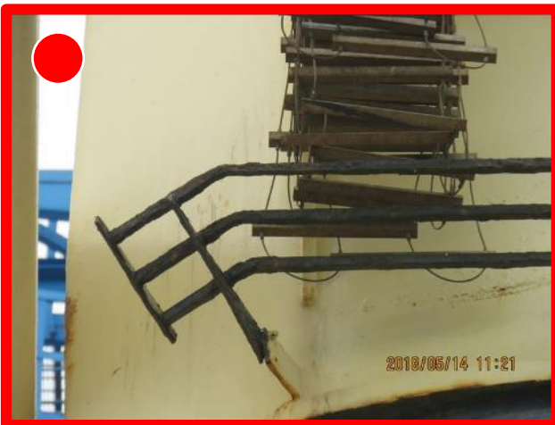
Wastage on emergency escape platform / grid
