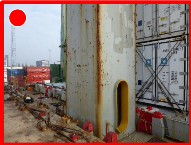
Excessive corrosion along pedestal
