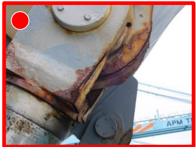
Excessive corrosion on jib mounting point
