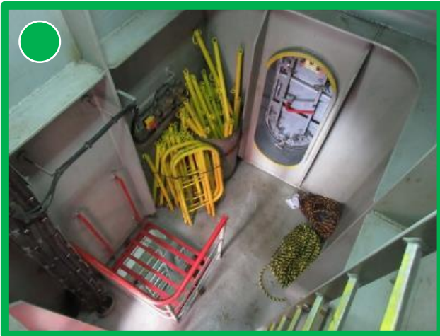
Pedestal entrance, some stored items but not obstructing (passage to ladder is free)
